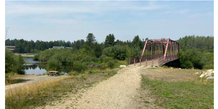
Sheep Bridge and Existing River Access
